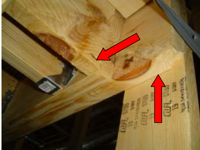
Band and joist no bearing on ends example
